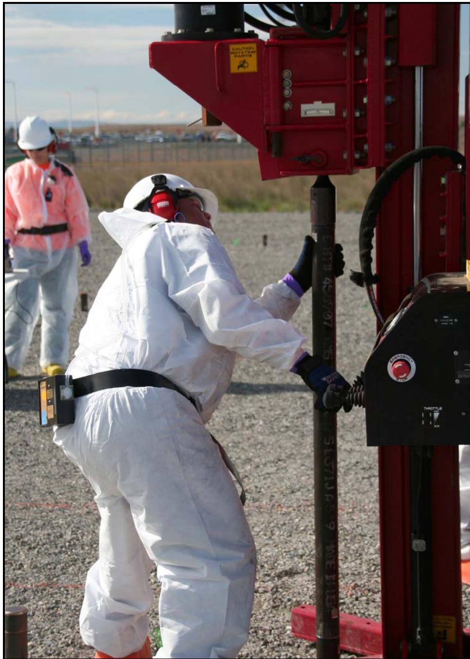
Cone penetrometers are installed to a depth of approximately 24 feet. (Photo 9)
