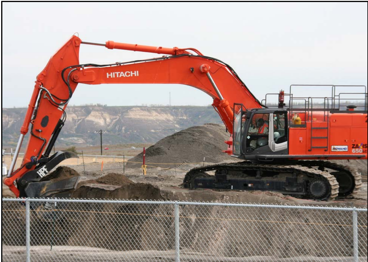
Washington Closure Hanford began trench excavation at the 618-10 Burial Ground. (Photo 4)
