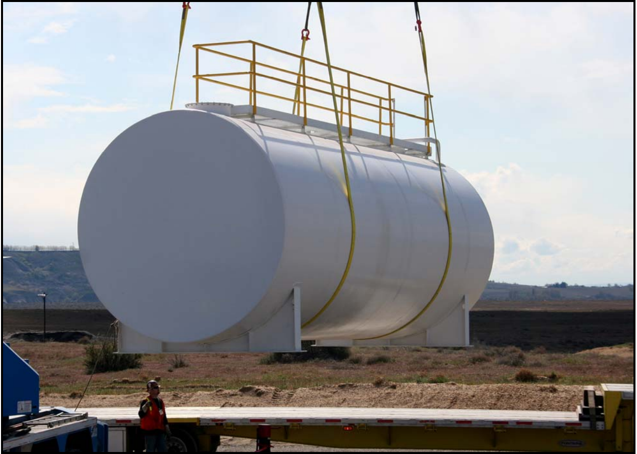
Each of the water tanks used for dust suppression at the 618-10 Burial Ground has a capacity of 22,000 gallons. (Photo 8)
