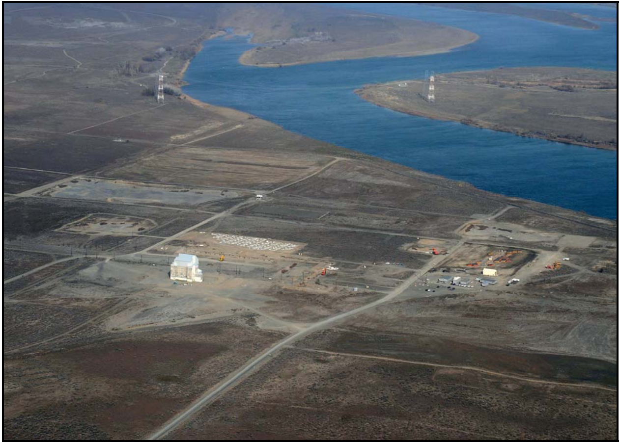
An aerial view from the southeast shows 100-F Area, where Recovery Act dollars are funding the remediation of 19 waste sites. (Photo 7)
