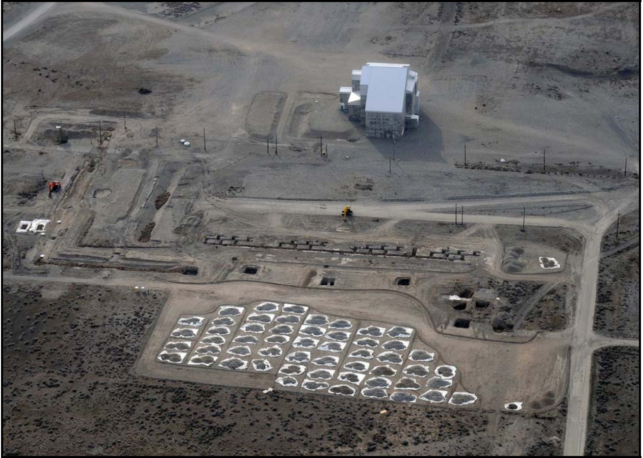
An aerial view from the east side of F Reactor shows material from the test pit campaign at 100-F-57 that was placed on white plastic. (Photo 8)
