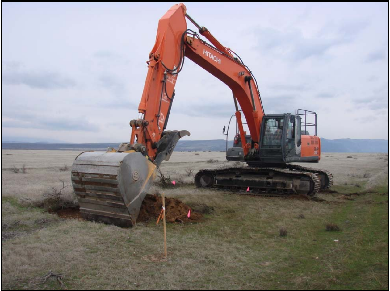
Remediation was completed this week at five IU 2 & 6 waste sites.
