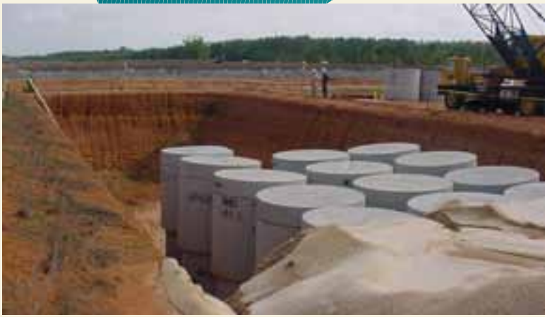
This LLW disposal site accepts waste from States participating in a regional disposal agreement.
