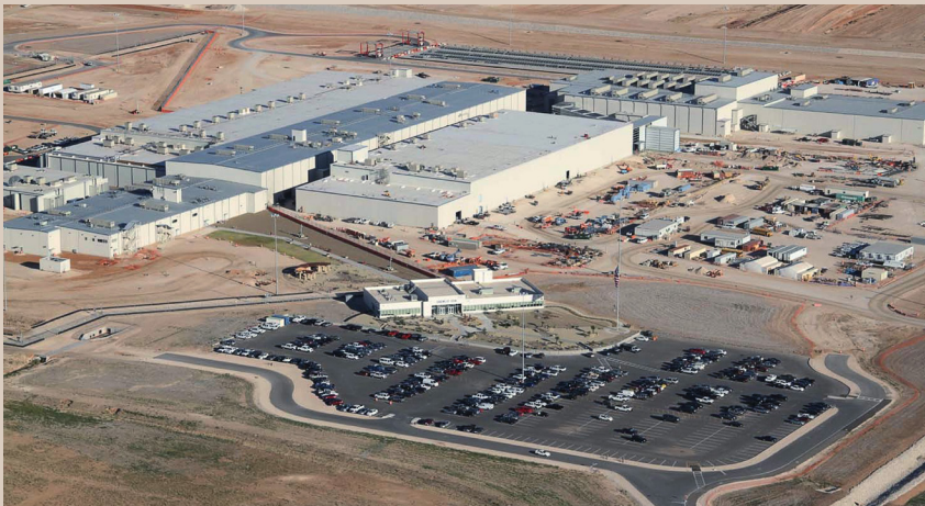
URENCO USA gas centrifuge uranium enrichment facility in Eunice, NM.
