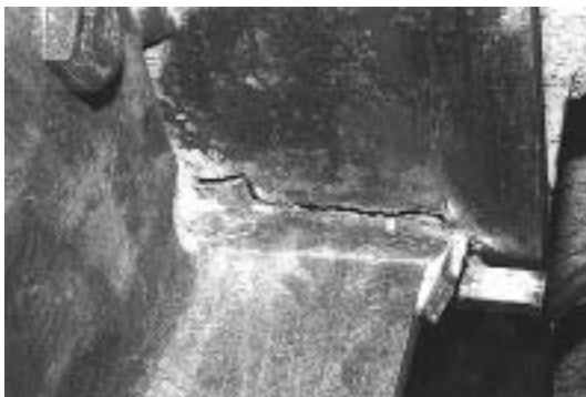
a. Fracture at Fused Zone
