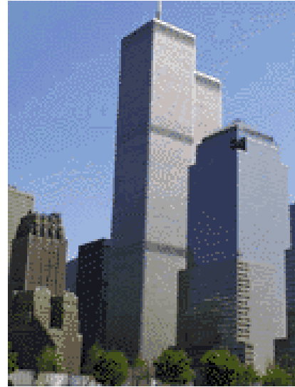
Many of the tallest buildings in our major cities are of WSMF construction.
