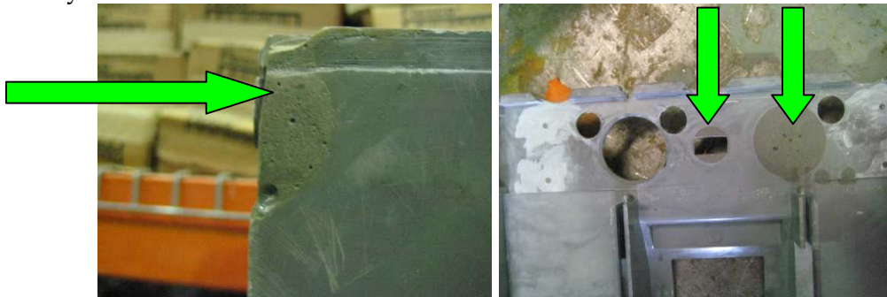
Epoxy Repair to Case Corner
