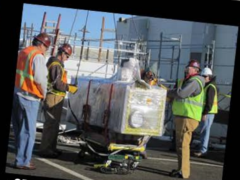
GB HC-11 on a Lift Table Being Prepared by Riggers to be loaded into SLB2
