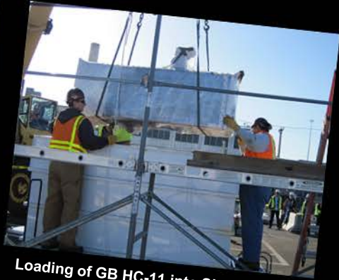
GB HC-11 on a Lift Table Being Prepared by Riggers to be loaded into SLB2
