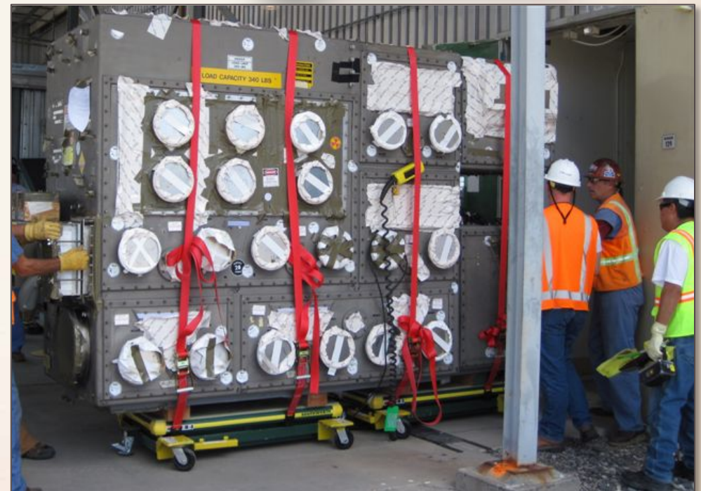
Glovebox removal from Plutonium Process Support Laboratory area
