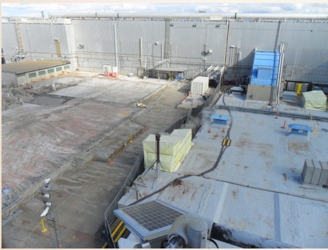
Demolition of PFP Vault Building
