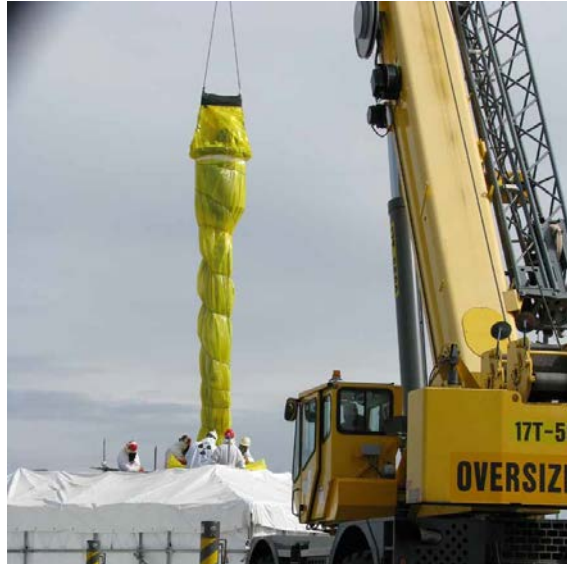
AN-106 Pump Successfully Removed in March - Retrieval activities in C-107 continue
