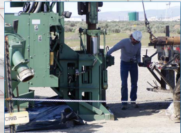
Pushing with Diesel Hammer
