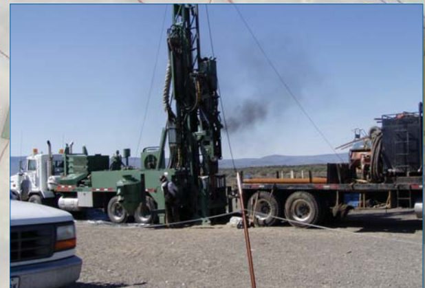
Diesel Hammer Push Technique
