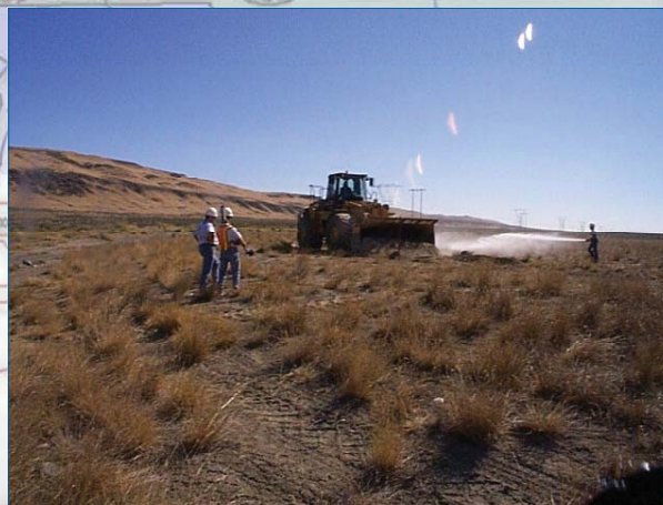
Preparing Site for Test Pit
