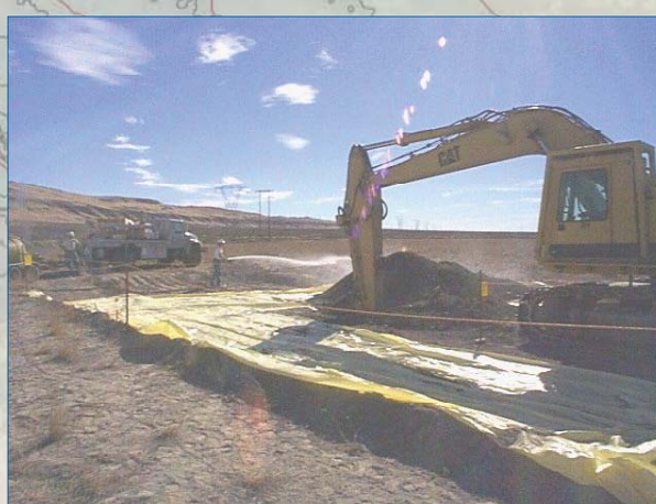
Excavating Test Pit
