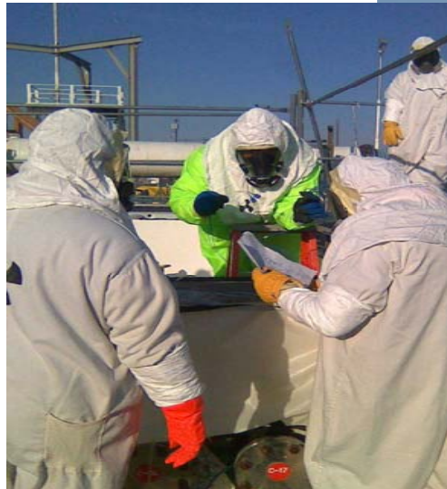
Crews installed thermocouples on waste transfer lines to improve temperature monitoring
