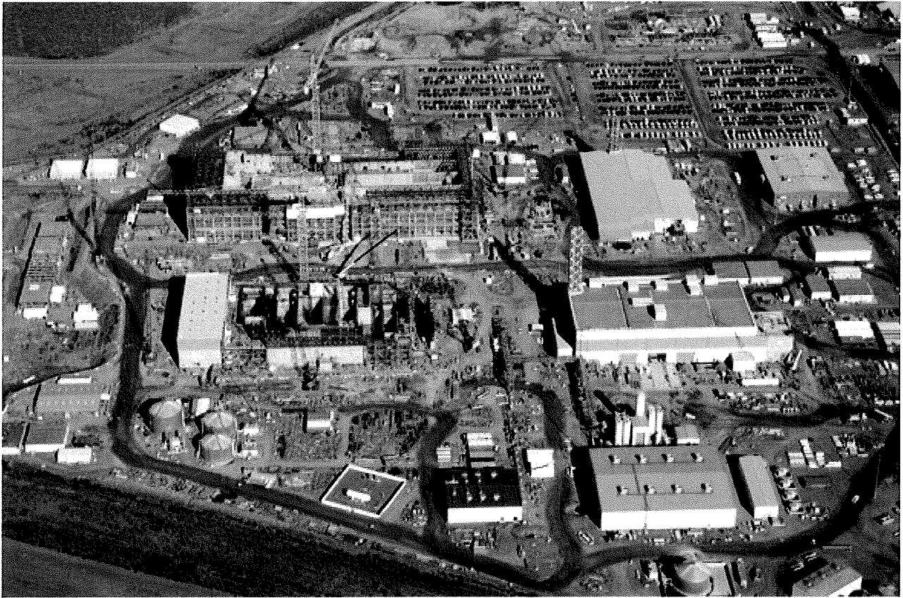
Figure 4-1. Waste Treatment and Immobilization Plant Construction Site, October 2011.
