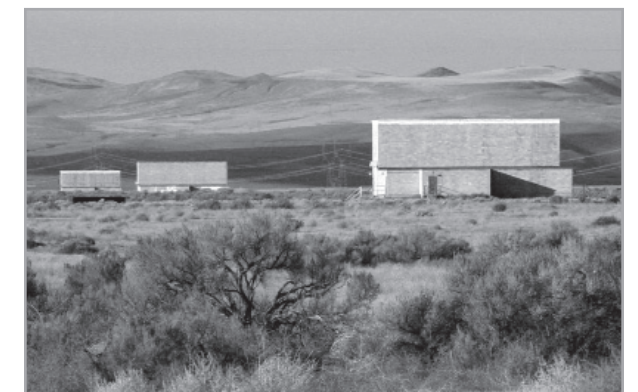
Building 212 N (foreground) was a nuclear facility that was demolished in 2009.
