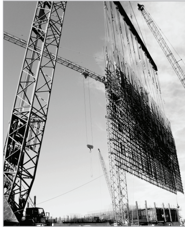
Cranes lift rebar and framework to the pretreatment facility at WTP.
