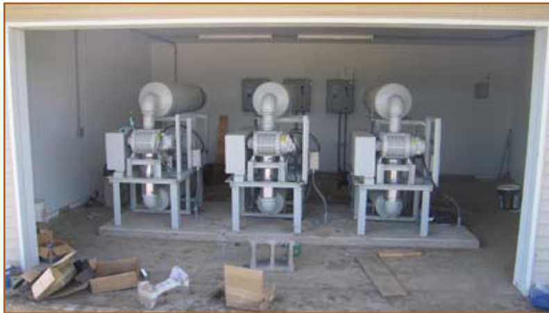
Figure 19: 18-foot x 24-foot blower building under construction.
