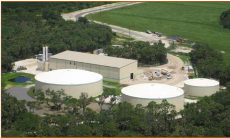
Figure 40: Aerial view of the newly constructed $30 million Brighton WTP owned and operated by the Seminole Tribe of Florida.
