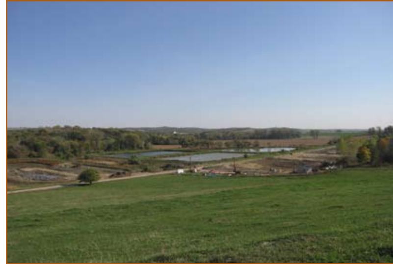
Figure 20: View of nearly completed project.
