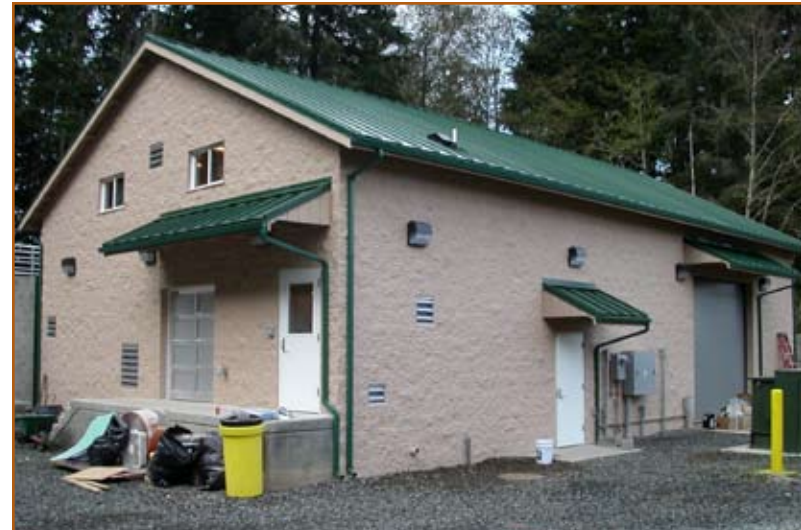
Figure 16: New Makah WTP near completion.
