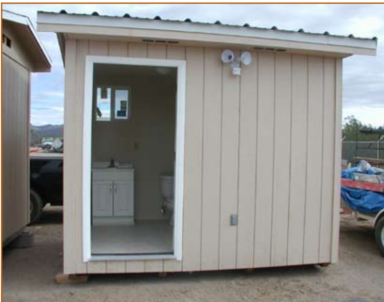
Figure 29: Staging area with front of bathroom.
