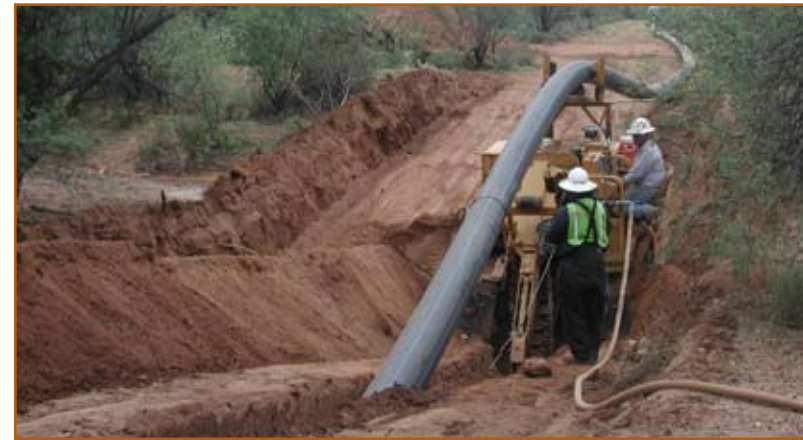
Figure 26: Installation of the watermain.
