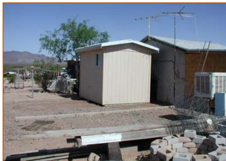
Figure 32: Finished and installed modular bathroom.
