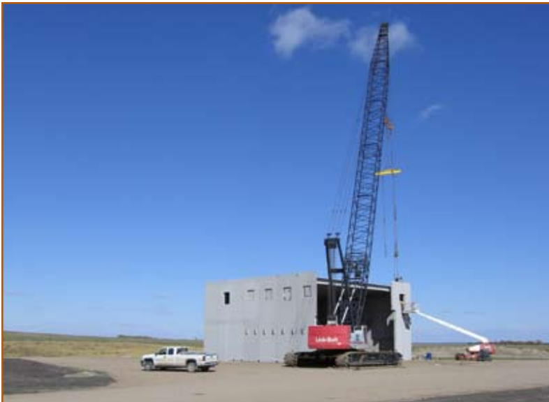
Figure 21: Setting pre-cast concrete wall panels for transfer station building.
