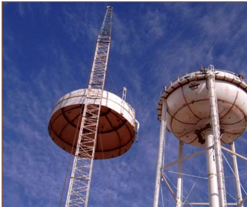
Figure 27: Construction of the elevated water storage tank.
