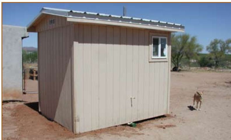
Figure 31: Back of modular bathroom.
