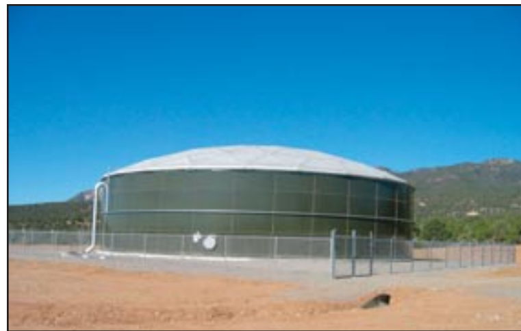
Figure 36: Completed 906,000 gallon water reservoir on the Ute Mountain Reservation, Colorado.
