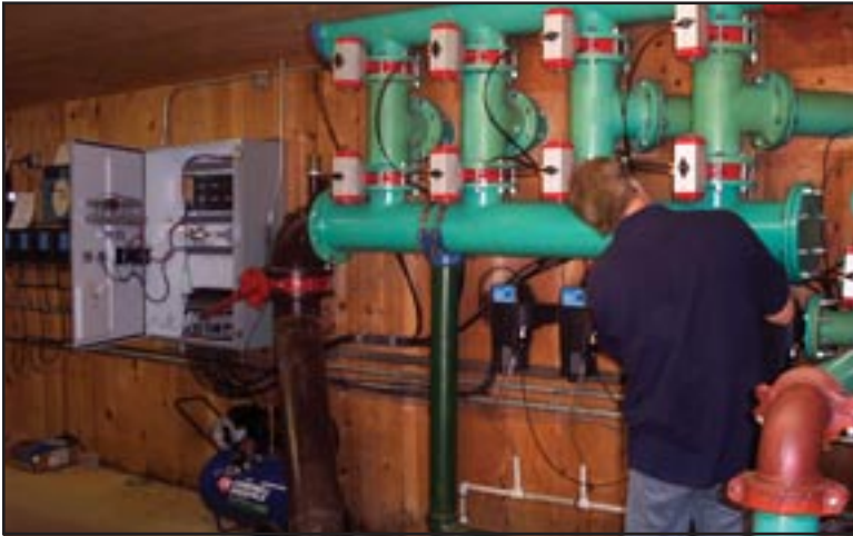
Figure 15: Contractor working on filter piping and controls in treatment building.
