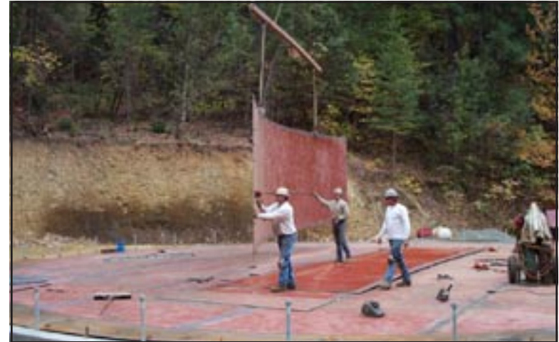
Figure 14: 1 million gallon water storage tank under construction.
