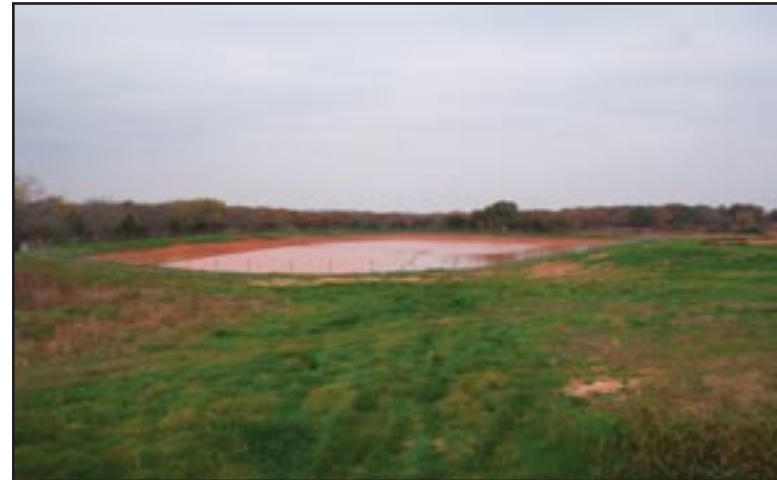
Figure 34: Completed lagoon with grass and fencing.
