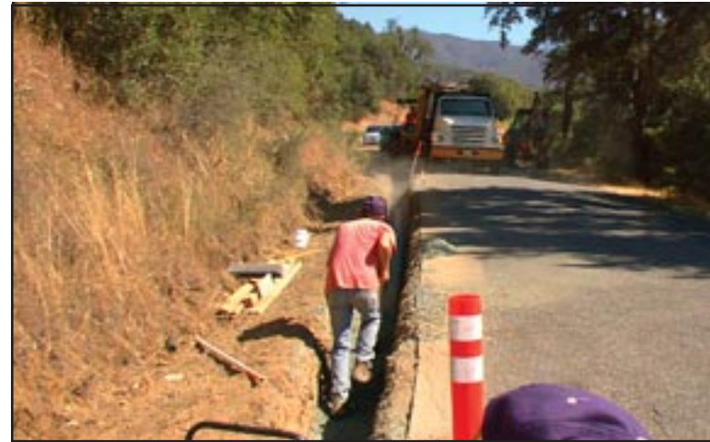
Figure 18: 8-inch PVC pipe installation with pipe embedment.
