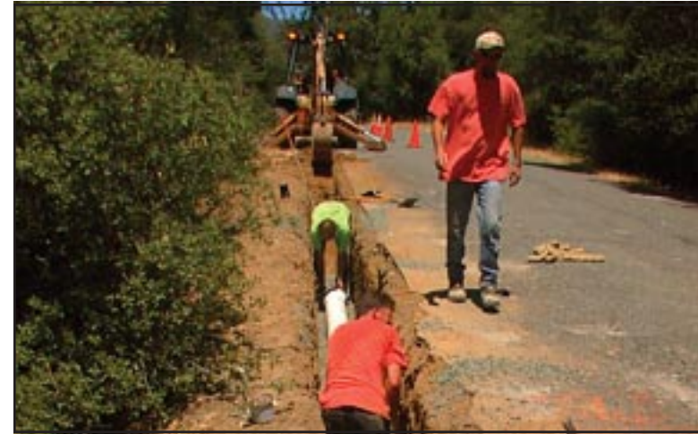
Figure 20: 8" PVC water installation.
