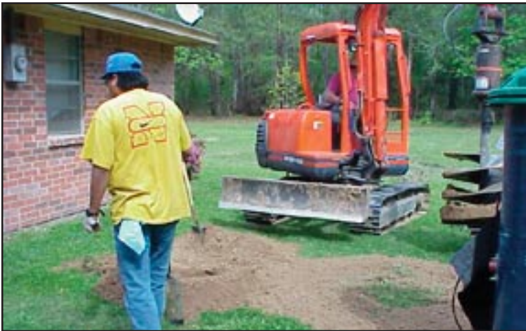
Figure 24: Tribal crew installing individual grinder lift station.
