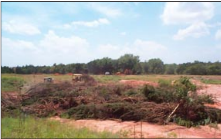
Figure 29: Clearing and grubbing lagoon site by Shawnee OEH force account crew.
