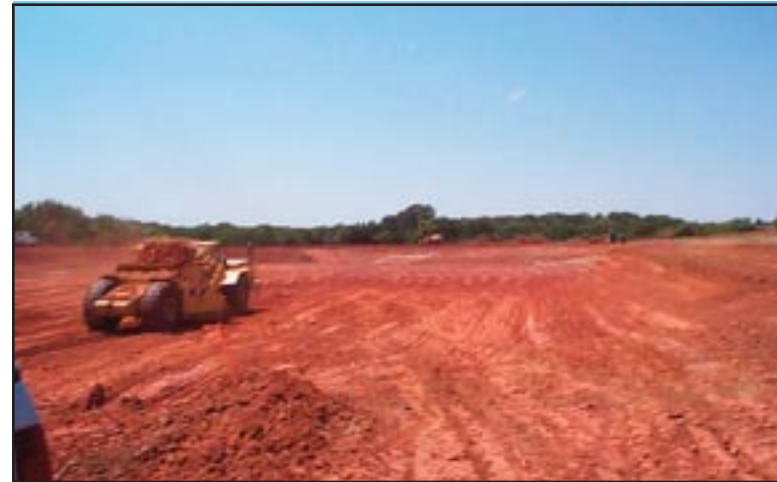
Figure 30: Initial excavation and berm compaction of lagoon.
