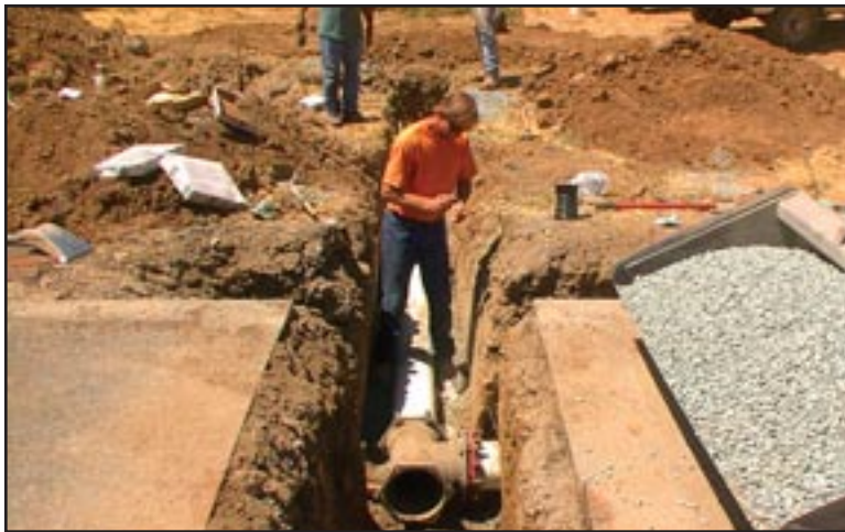
Figure 22: Contractor tying into the existing Dewell community water main.
