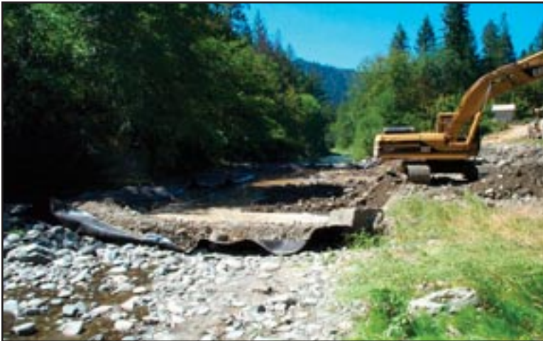
Figure 13: Initial cofferdam construction in Elk Creek.
