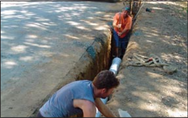
Figure 21: Contractor installing water main in Hardisty community.
