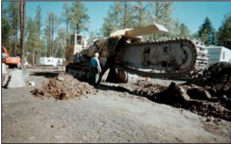
Figure 43: Rock trencher excavates a deep sewer main as part of a $10 million Hon Dah regional sewer project, Ft. Apache Reservation, Arizona.
