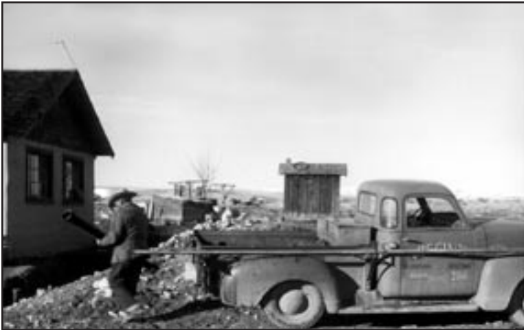
Figure 1: Construction of a septic system, 1960's
