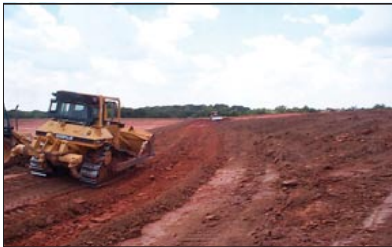
Figure 31: Placing topsoil on north lagoon berm.
