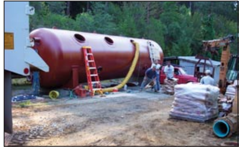
Figure 16: Filling the new 720 gallon-per-minute filter with filter media.
