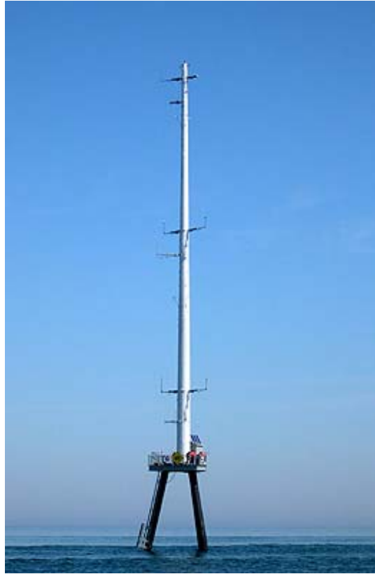
Figure 3.1. Cape Wind Meteorological Tower. (Source: Cape Wind Associates, LLC).
