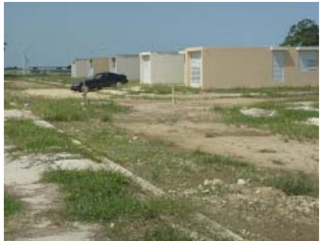
Partial view of houses under construction at Vilar Development project.
