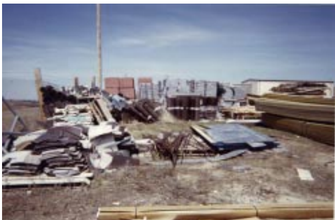
Materials and supplies haphazardly stored are exposed to the elements and vandalism.
