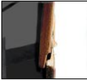
Split entry door trim.
