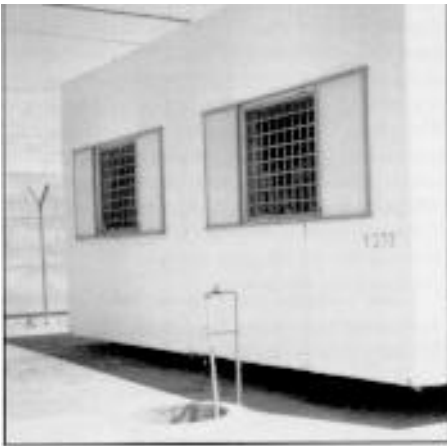
Isolation building, military prison camp Ketsiot.
