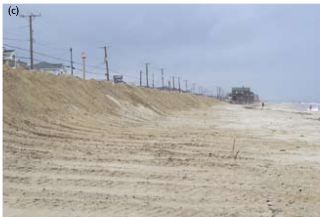
Figure 12.6 Retreat. (a) June 2002. Houses along the shore in Kitty Hawk, North Carolina. Geotextile sand bags protect the septic tank buried in the dunes. (b) October 2002. (c) June 2003 [Photo source: ©James G. Titus, used with permission].
