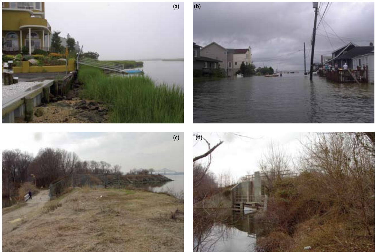
Figure 11.4 Vulnerability of New Jersey's coastal zone. (a) Wetland fringe lacks room for wetland migration (Monmouth, August 2003). (b) Low bay sides of barrier islands are vulnerable to even a modest storm surge (Ship Bottom, September 2, 2006). (c) Gibbstown Levee and (d) associated tide gate protect lowlying areas of Greenwich Township (March 2003) [Photo source: ©James G. Titus, used with permission].
