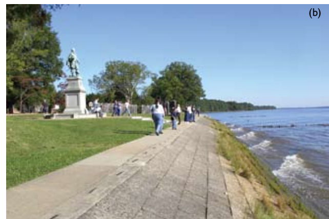
Figure 6.3 Two types of stone revetments (a) near Surfside, Texas (May 2003) and (b) at Jamestown, Virginia (September 2004) [Photo source: ©James G. Titus, used with permission].
