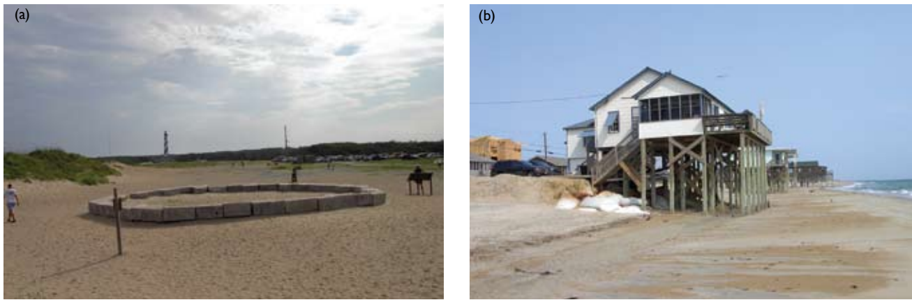
Figure 6.8 Relocating structures along the Outer Banks (a) Cape Hatteras Lighthouse after relocation at the Cape Hatteras National Seashore, Buxton, North Carolina (June 2002); the original location is outlined in the foreground, and (b) a home threatened by shore erosion in Kitty Hawk, North Carolina (June 2002) The geotextile sand bags are used to protect the septic system [Photo source: ©James G. Titus, used with permission].
