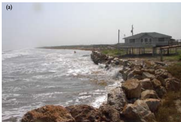
Figure 6.3 Two types of stone revetments (a) near Surfside, Texas (May 2003) and (b) at Jamestown, Virginia (September 2004) [Photo source: ©James G. Titus, used with permission].
