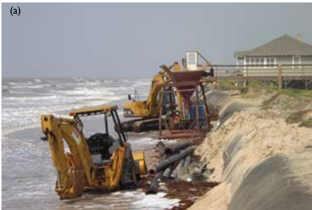
Figure 6.2 Geotube (a) before and (b) after being buried by beach sand at Bolivar Peninsula, Texas (May 2003) [Photo source: ©James G. Titus, used with permission].
