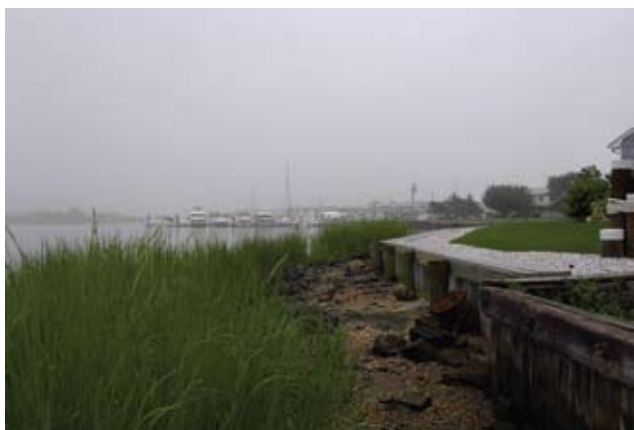
Figure 5.2 Fringing marsh and bulkhead, Monmouth County, New Jersey (August 2003) [Photo source: ©James G. Titus, used with permission].
