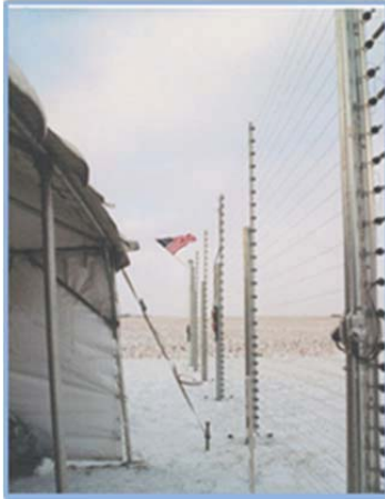
Construction of the non-lethal/lethal fence systems at USPs is nearing completion; five projects remain. Systems can operate in three modes: stun, non-activated stand-by, or watch.
