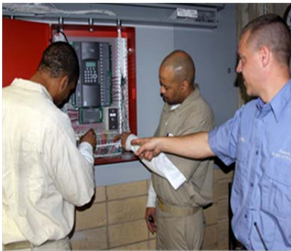
L: Air handler
