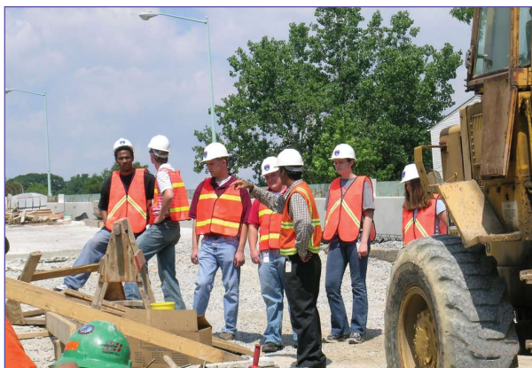
Co-op students at Taylor Street Bridge Replacement, DC BH-3202(8), Washington, District of Columbia (District Department of Transportation)
