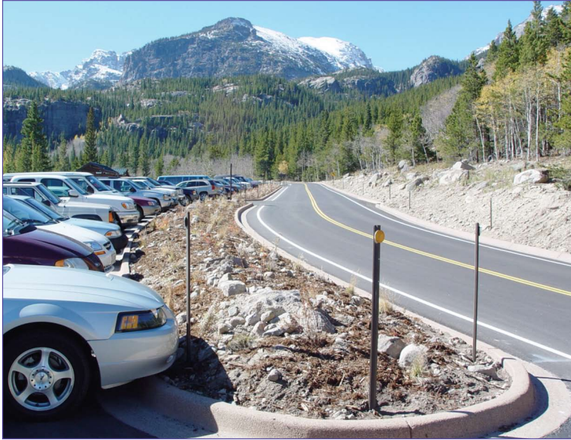
Relocation of parking areas increases safety and decreases environmental impacts. Bear Lake Road, Rocky Mountain National Park, Colorado (National Park Service)
