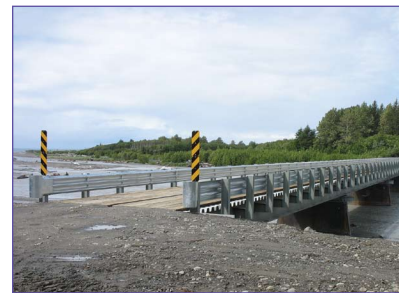
Yakataga Bridge Replacement, Yakutat Borough, Glen Allen, Alaska (Bureau of Land Management)
