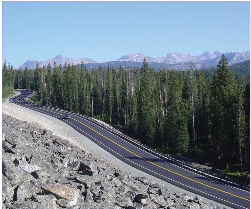
Beartooth Highway Emergency Repairs, Yellowstone National Park, Cooke City, Montana (National Park Service)
