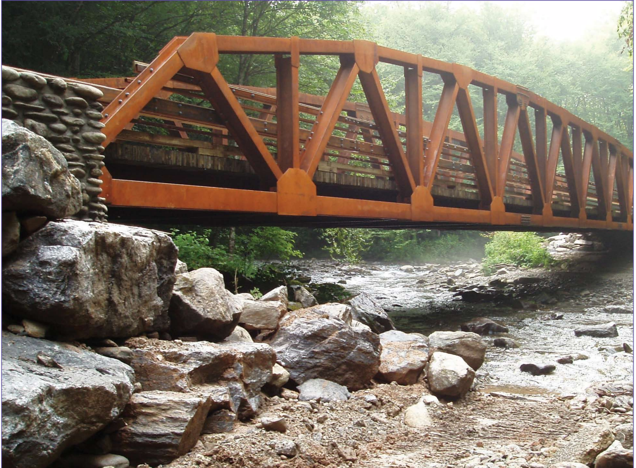
Straight Fork Bridge Profile, Great Smoky Mountains National Park, Swain County, North Carolina (National Park Service)
