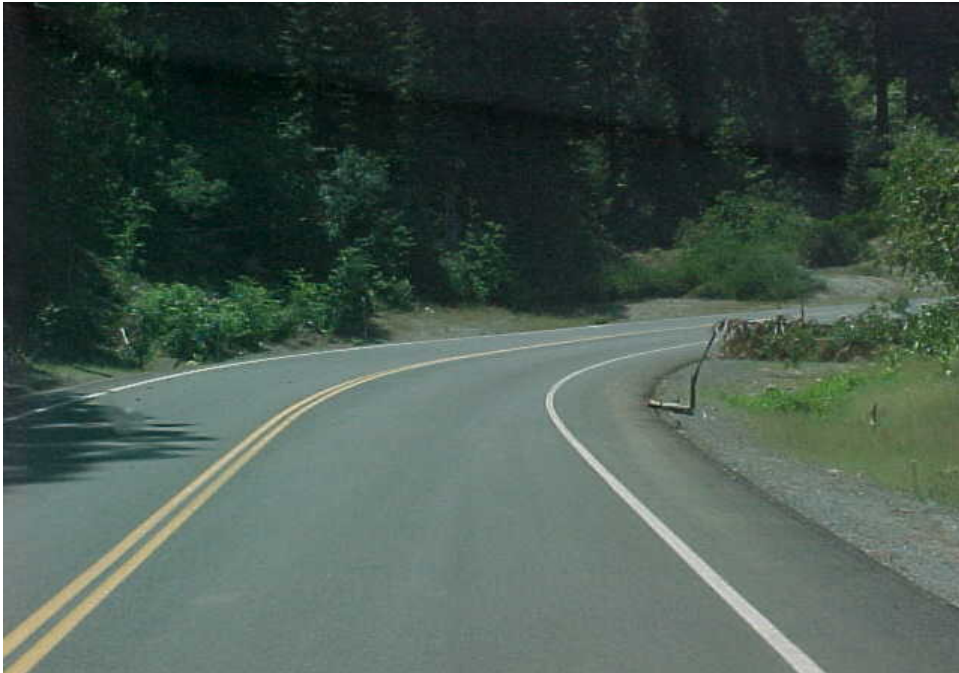
Incorrect striping at curve widening area. Place the centerline striping midway between the edges of the widened travel way. In other words, the distance from the edge of pavement to the edgeline should remain constant along the travel way.
