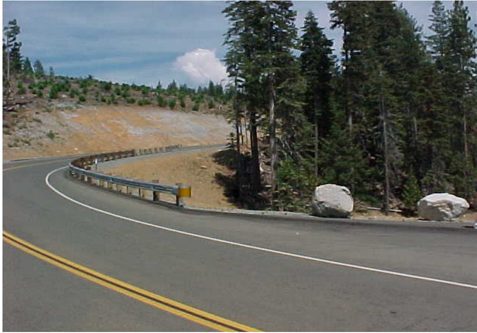
Guardrail improvements could have been made by extending the rail.
