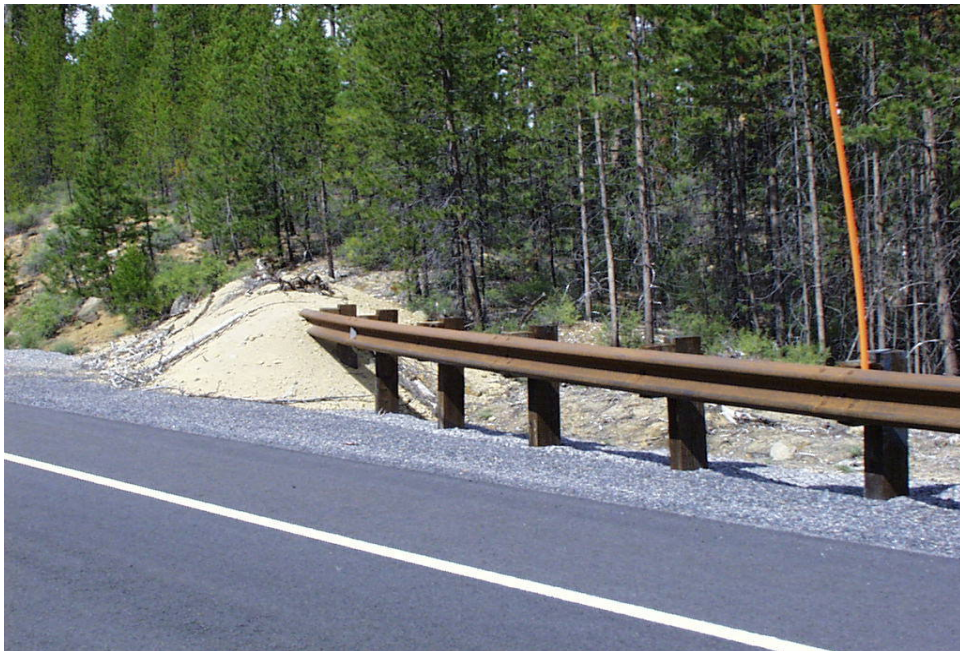
Terminating the barrier beyond the clear zone with earth berm is desirable provided the roadway and terrain are suitable. Care should be taken not to make the berm a hazard.
