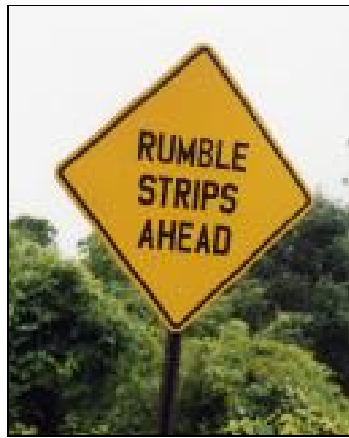
Warning Sign used in advance of initial shoulder rumble strip installation
