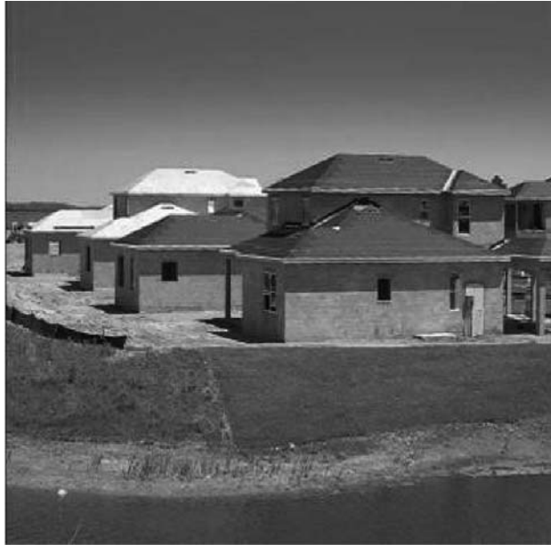
Figure 6. A typical new, residential construction work site.
