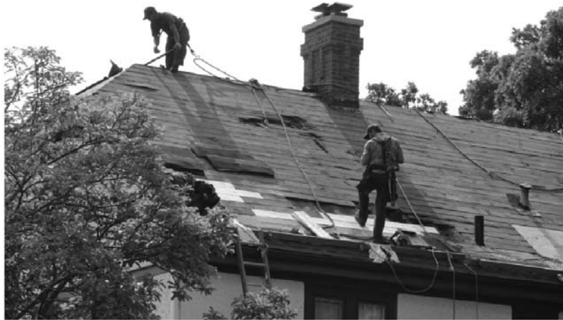
Figure 5. Workers in PFAs on a 10:12 pitched roof.
