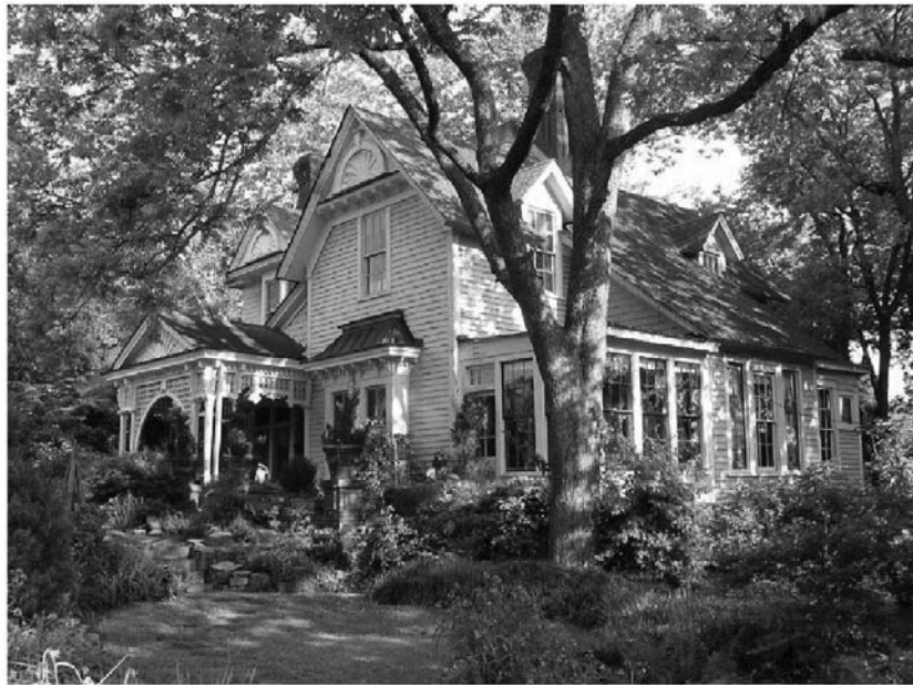
Figure 7. Site issues on a typical residential reroofing project.
