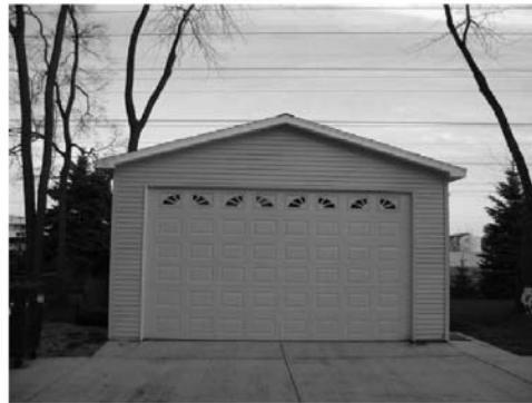
Figure 3. Garage with 4:12 pitched roof.
