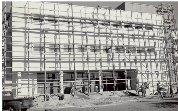
Construction of HQ USAFSS, Entrance Bldg 2000, 1953
