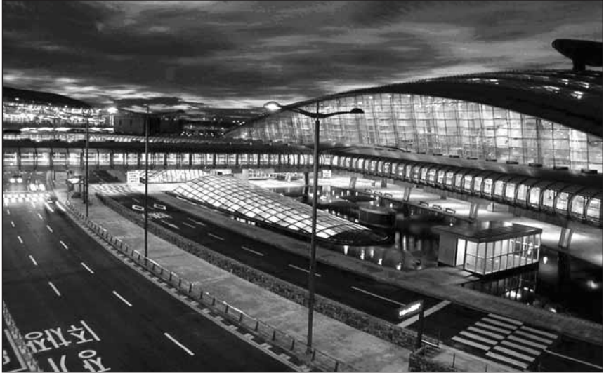
Incheon International Airport
