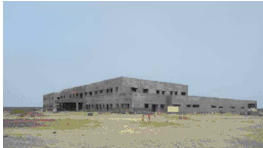
The Missan Surgical Hospital under construction in Missan province. (USACE photo)
