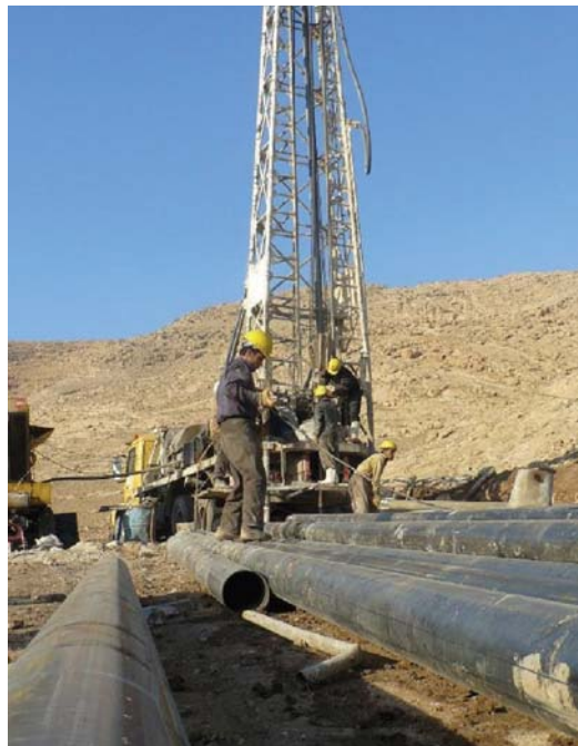
Workers in Iraq drill a drinking-water well. (USAID photo)
