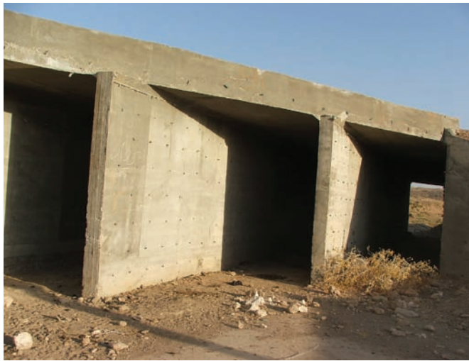
Site Photo 11. Box culverts for new road.
