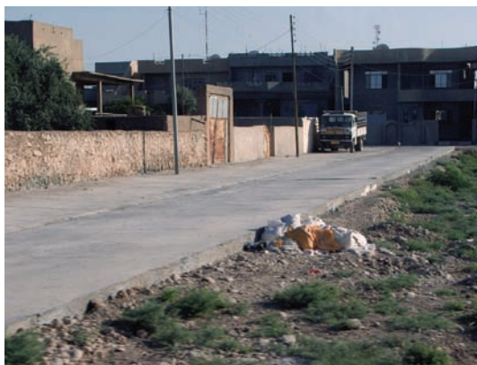
Site Photo 14. Newly constructed road.
