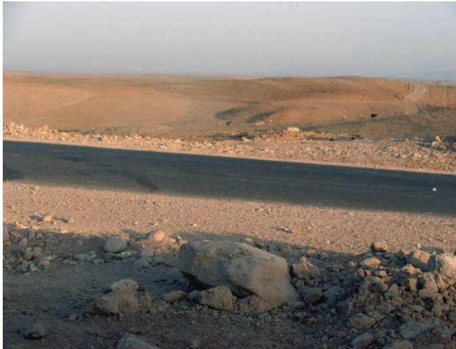
Site Photo 10. Newly constructed road with shoulders.
