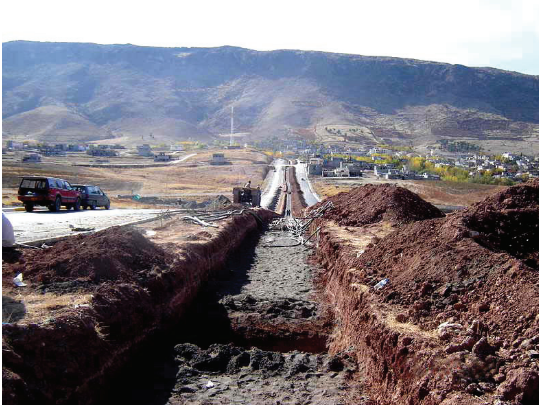
CERP-funded road construction.
