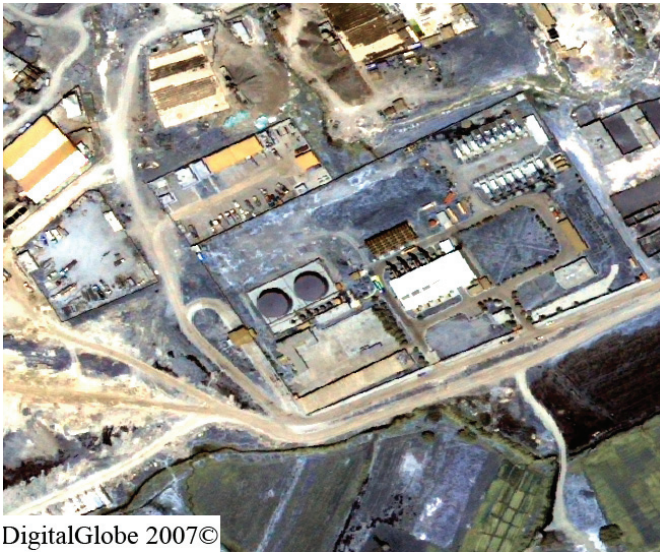
Aerial Image 1. Imagery overview of the Shasheed Shazad Power Plant taken on July 6, 2007.
