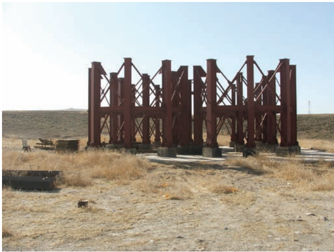
Site Photo 2. View of the partially constructed stationary silos.
