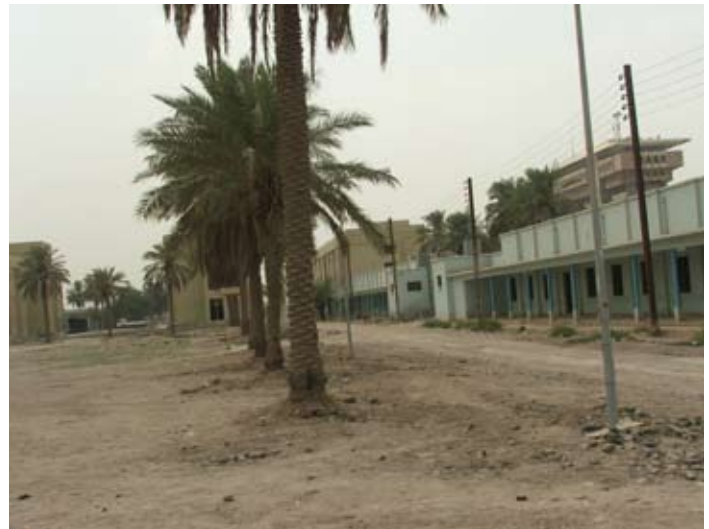
Site Photo 29. Existing barracks at the Baghdad Police College.
