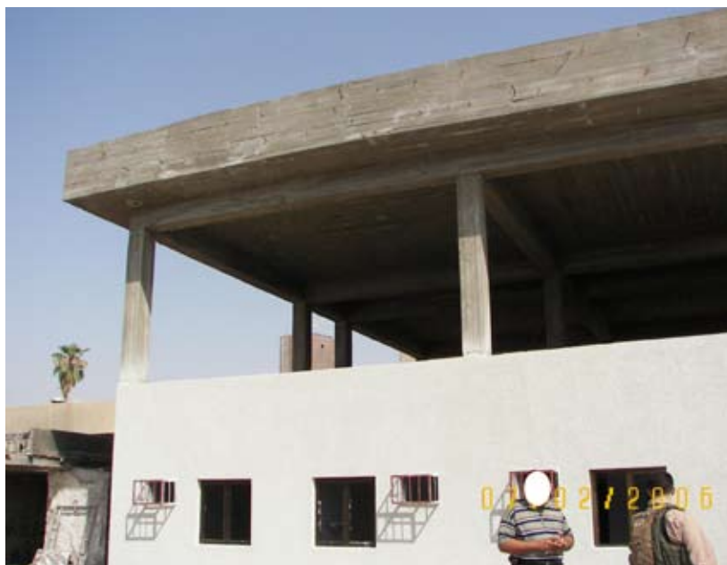
Site Photo 3. First-floor columns and beams supporting roof.
