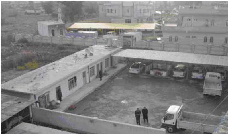
Site Photo 18. Contractor delivered generator (bottom left), but never connected and load tested it.
