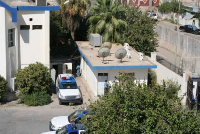
Site Photo 17. Only two (left rear edge of rooftop) of six split-unit air conditioners required were installed in the new reception center.
