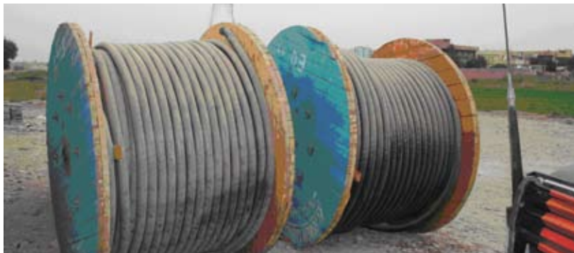
Site Photo 21. 3 X 150 mm 2 electrical cable supplied on rolls 503 m long. (Photo provided by USACE)
