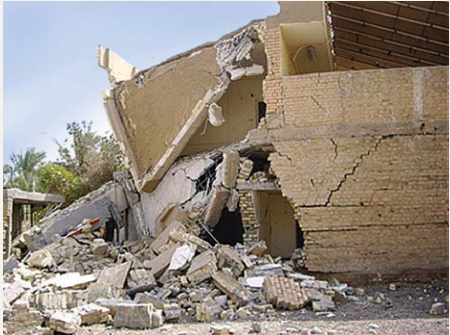
Damage inflicted by a rocket on the house across the street from Judge Radhi’s residence in the International Zone, summer 2007. (Former DoS official photo)
