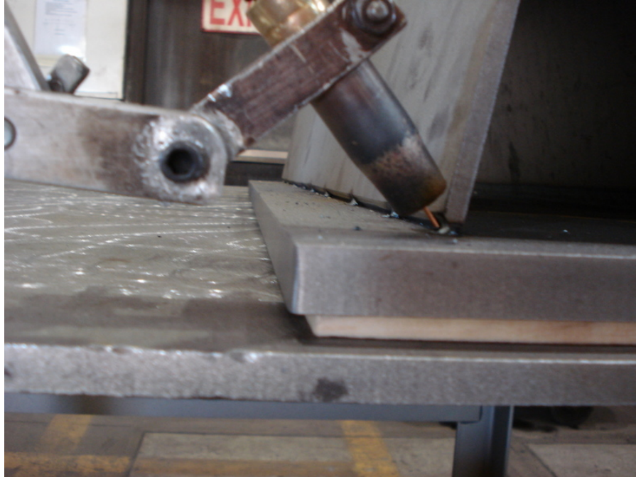
Figure 7-8 Wire Angles and Diameter are Critical for Suitable Rib-to-deck Welding. The Picture shows a Demonstration Piece with the Wire Size and Angle Prepared
