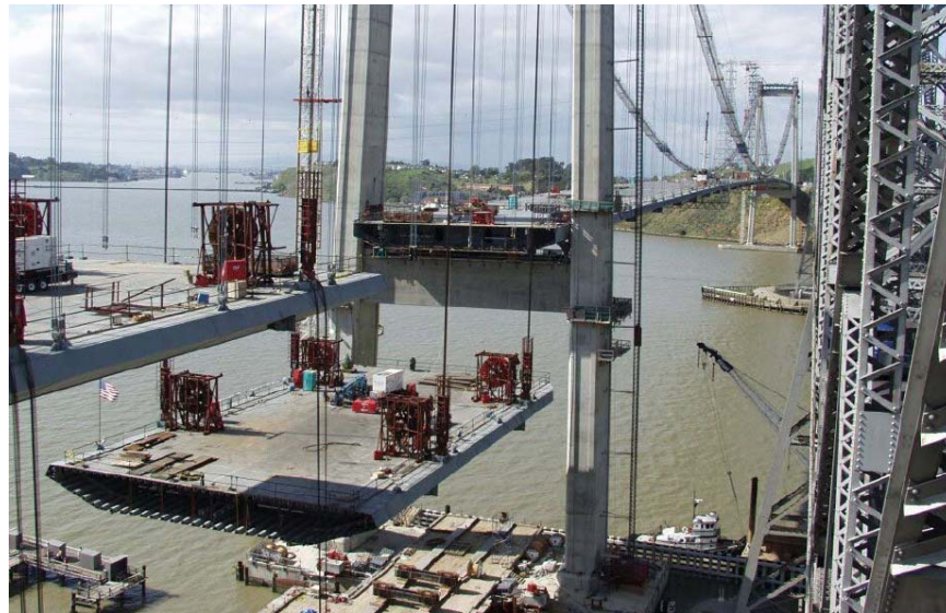
Figure 1-2 Erection of Orthotropic Box Girder Segment for the Alfred Zampa Memorial Bridge lifting a Deck Segment into Place
