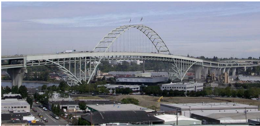
Figure 2-3 Photo of the Fremont Bridge over the Willamette River in Portland, OR. The Upper Deck is an Orthotropic Steel Deck for the Full Length of the Main Span Unit.
