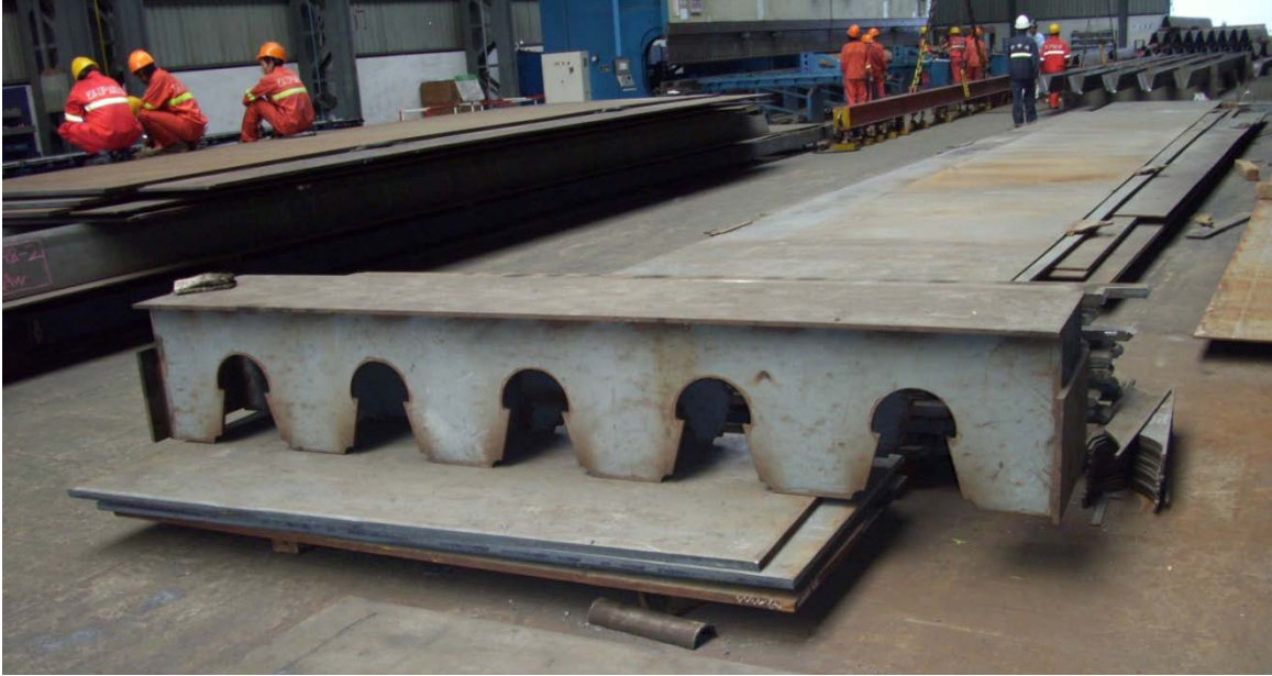
Figure 7-9 Fabricators use Jigs Such as the One Shown to Help Achieve Proper Alignment in the Ribs
