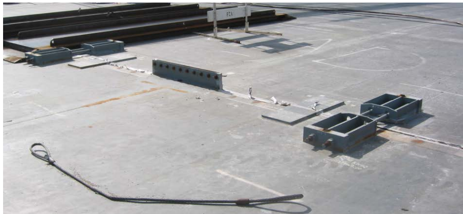
Figure 7-15 Temporary Fit-Up Lugs are Necessary for OD Construction. Tensioning Rods Bridge Two Sections to Pull Together and Align the Adjacent Panels
