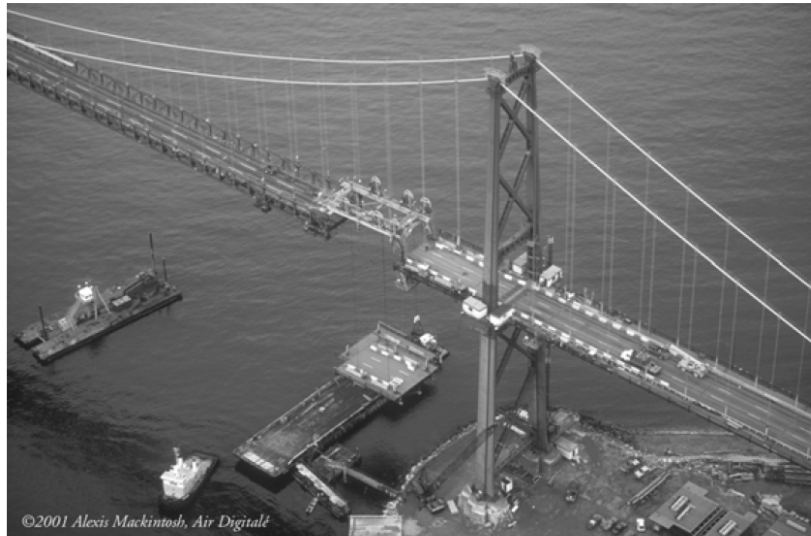
Figure 2-4 Aerial Photo of the Lions Gate Bridge showing the Redecking with Orthotropic Deck Segments being Lifted into Place
