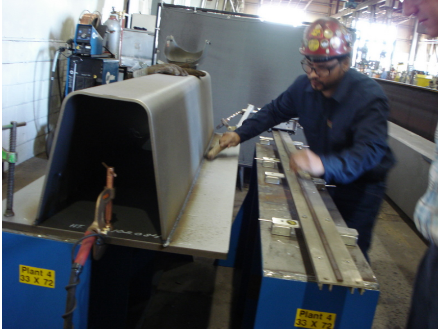
Figure 7-6 The Fabricator will Develop a Procedure for Rib-to-Deck Welding as the Worker in the Photo is Testing
