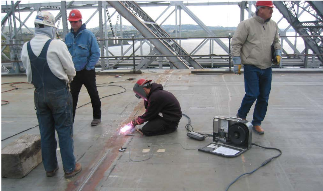
Figure 7-14 Field Welding of the Transverse Deck Plate Joint during Construction
