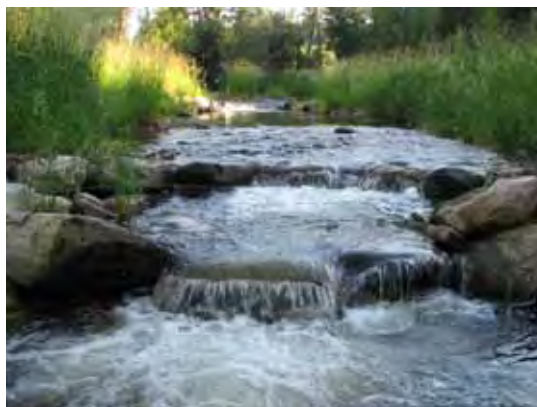
Figure 2. The old push-up diversion dam was replaced with a series of three boulder weirs that allow upstream passage for adult and juvenile fish.
