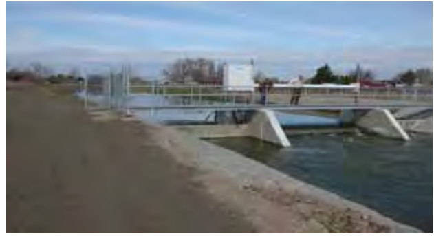
Figure 2. New automated check controlled from SVID office, reduces operational spills and can be adjusted remotely.
