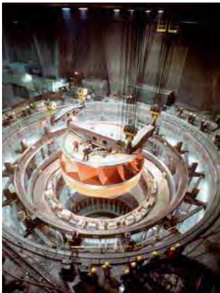
Photo: Third Powerhouse turbine runner being installed in 1974. Turbines are 16'8" in diameter, weigh approximately 1 million pounds each, and produce up to 805 megawatts of power.
