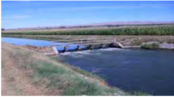
Figure 1. Picture of a manual check structure used to control water elevation are dangerous to adjust and labor intensive.
