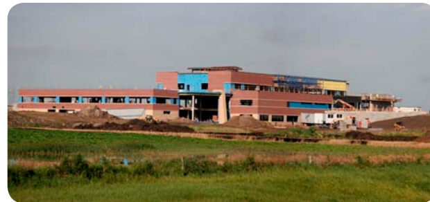
Jamestown Regional Medical Center under construction.
