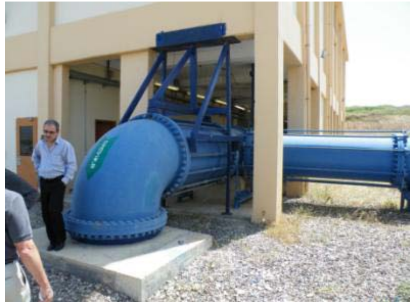
Site Photo 9. Steel brace connected to pump station building
