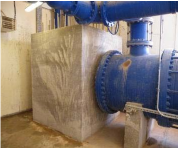
Site Photo 8. Concrete reaction block
