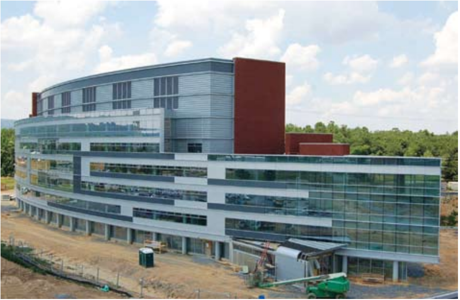
The National Biodefense Analysis and Countermeasures Center under construction.
