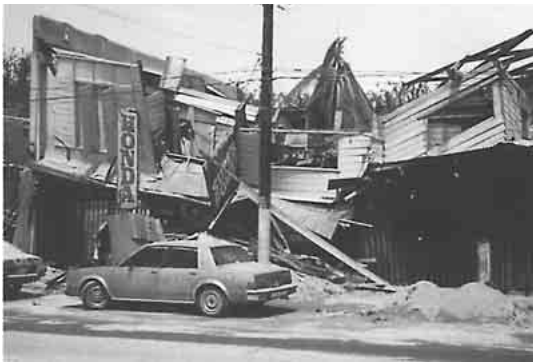
Following Mount Pinatubo's cataclysmic June 15, 1991, eruption, thousands of roofs collapsed under the weight of ash made wet by heavy rains (see example in photo above). Ash deposits from the eruption have also been remobilized by monsoon and typhoon rains to form giant mudflows of volcanic materials (lahars), which have caused more destruction than the eruption itself (photo at right shows village buried by lahars). (Photo above courtesy of Peter Baxter, University of Cambridge.)
