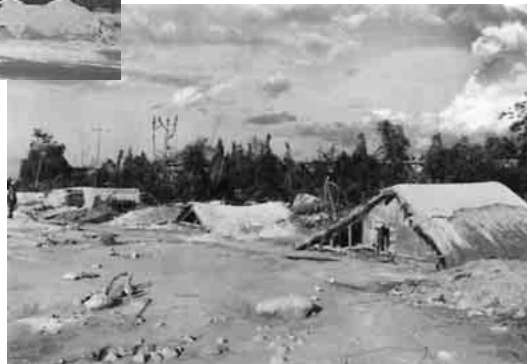
Following Mount Pinatubo's cataclysmic June 15, 1991, eruption, thousands of roofs collapsed under the weight of ash made wet by heavy rains (see example in photo above). Ash deposits from the eruption have also been remobilized by monsoon and typhoon rains to form giant mudflows of volcanic materials (lahars), which have caused more destruction than the eruption itself (photo at right shows village buried by lahars). (Photo above courtesy of Peter Baxter, University of Cambridge.)
