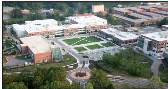
ORNL is located in Oak Ridge, Tennessee.
