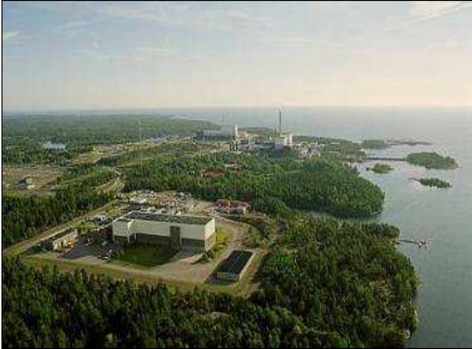
Figure 11. The Clab Interim Spent Fuel Storage Facility at Oskarshamn, Sweden.
