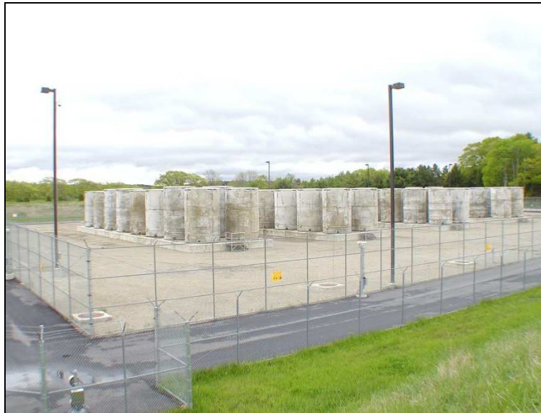
Figure 3. Dry Cask Storage Facility at the Decommissioned Maine Yankee Reactor Site
