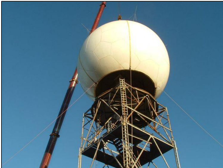
The dome being lifted off the old tower
