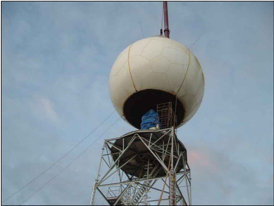
Dome being placed on the new tower
