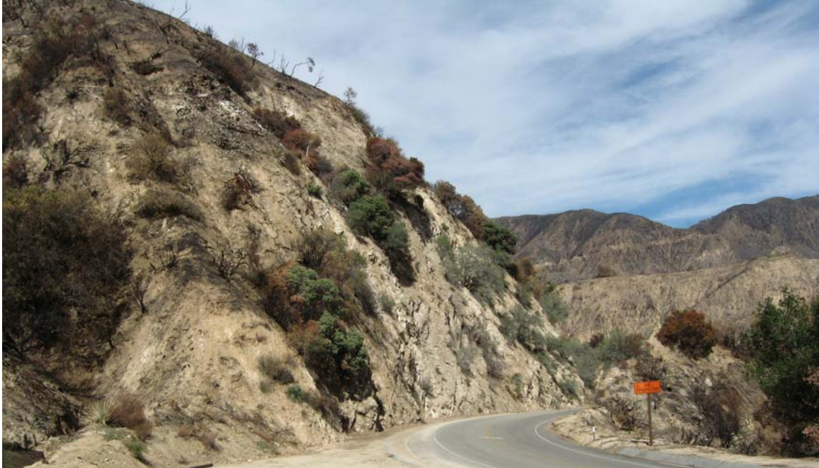
Photograph 3. Looking north along S.R. 2 (Angeles Crest Highway). Southern edge of original Station Fire perimeter on ridge to left. During the early morning hours of August 27, 2009, down canyon winds carried embers from this ridge to unburned vegetation on the downhill (east) side of S.R. 2 to the right. Photo taken on October 21, 2009.
