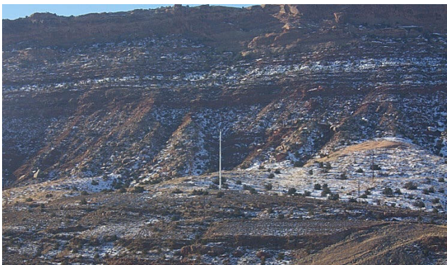
This is an untreated cellular tower viewed from Arches National Park.
