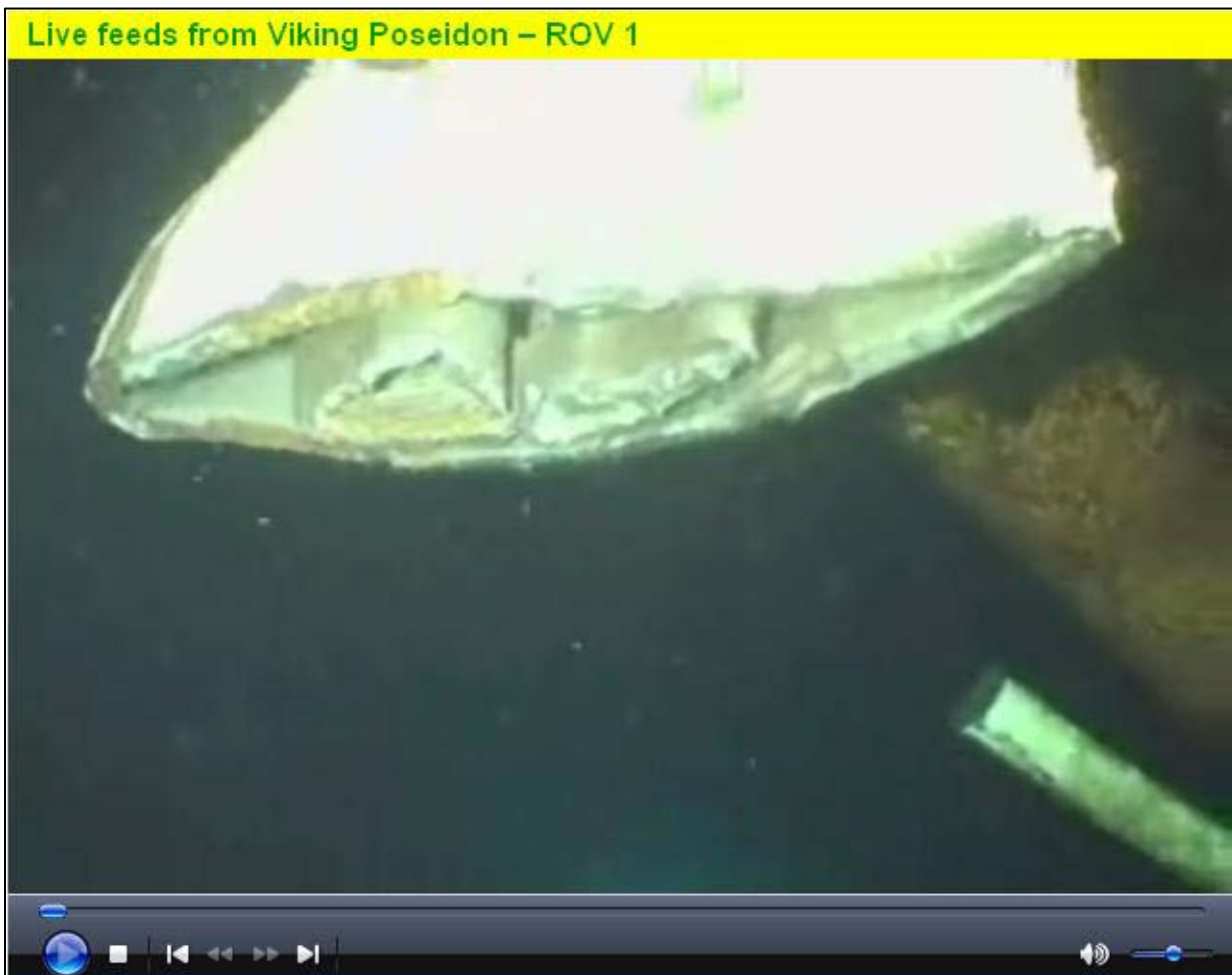
Figure 5: Cut Riser Showing Two Pipes Inside
