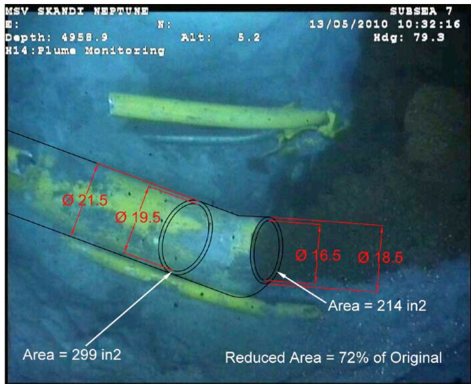
Figure 2: Riser Outlet Showing Its Reduced Cross-Sectional Area
