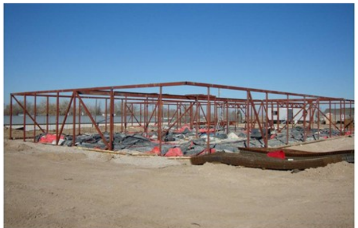
Frame of the new building
