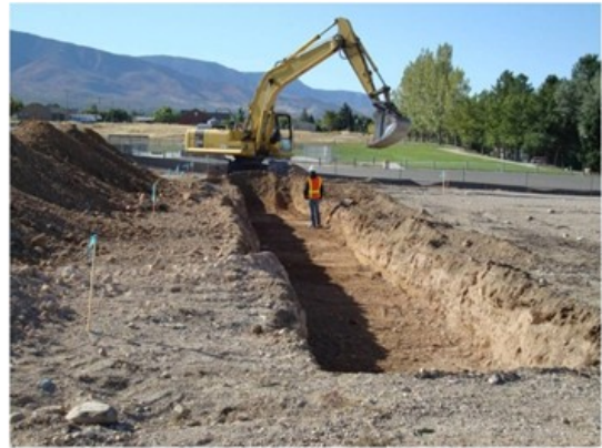
Digging the trench for the foundation
