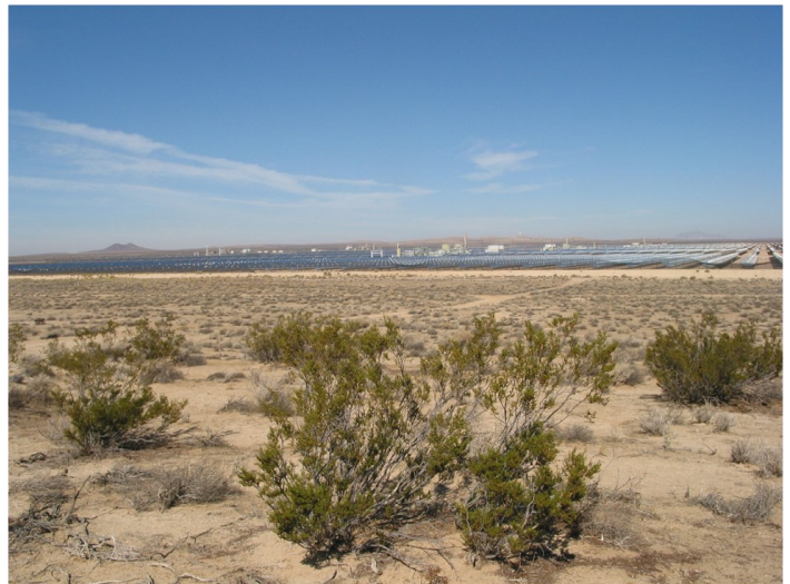
View of solar energy generating system on private land in Calif. Similar technology could be used on public lands. (H. Hartmann. Argonne)
