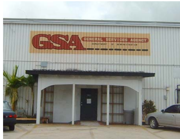
External view of GSA fronting Marine Corps Drive in Piti.
